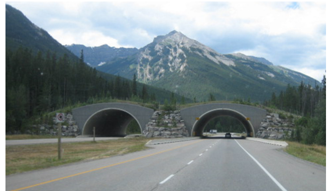
Figure 1. Wildlife Crossing, Alberta, Canada.
