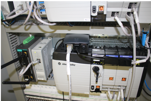
Figure 6: Raspberry PI placement on top of a PLC
